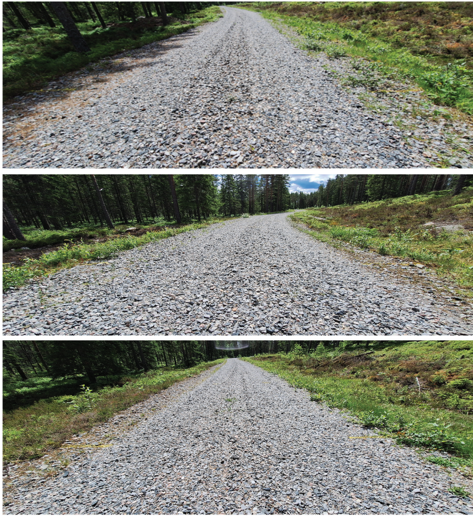
Figure 14. Visual inspection of section 1 (with stone mattresses) in Grängesberg. Photos: Andreas Waldemarson, VTI.
