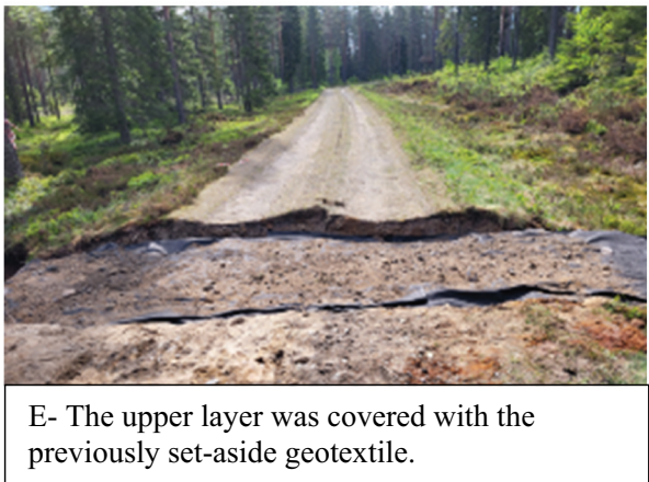
Figure 4. Field construction of stone mattresses. Photo: Johan Persson, Kopparfors.
