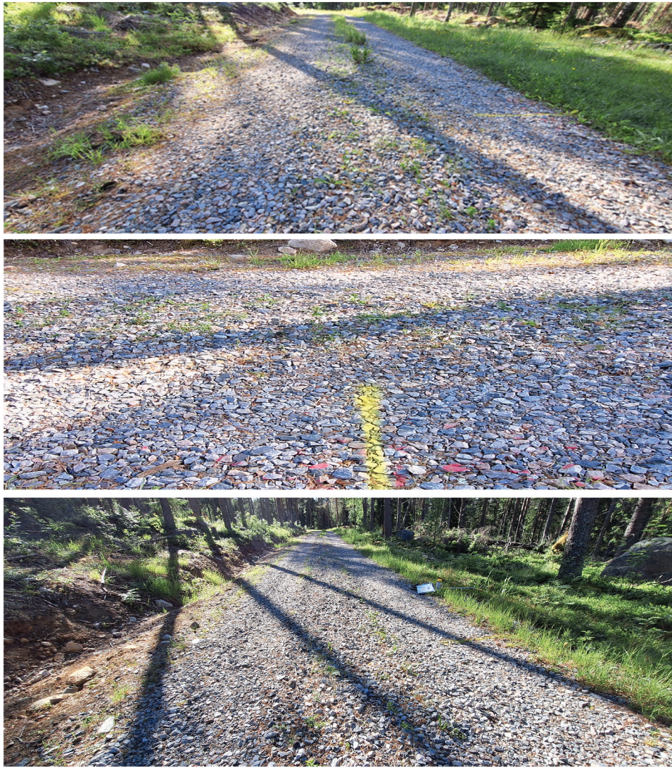
Figure 16. Visual inspection of section 2 (with stone mattresses) in Grängesberg. Photos: Andreas Waldemarson, VTI.
