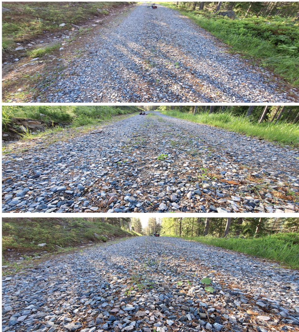
Figure 17. Visual inspection of section 2 (without stone mattresses) in Grängesberg. Photos: Andreas Waldemarson, VTI.
