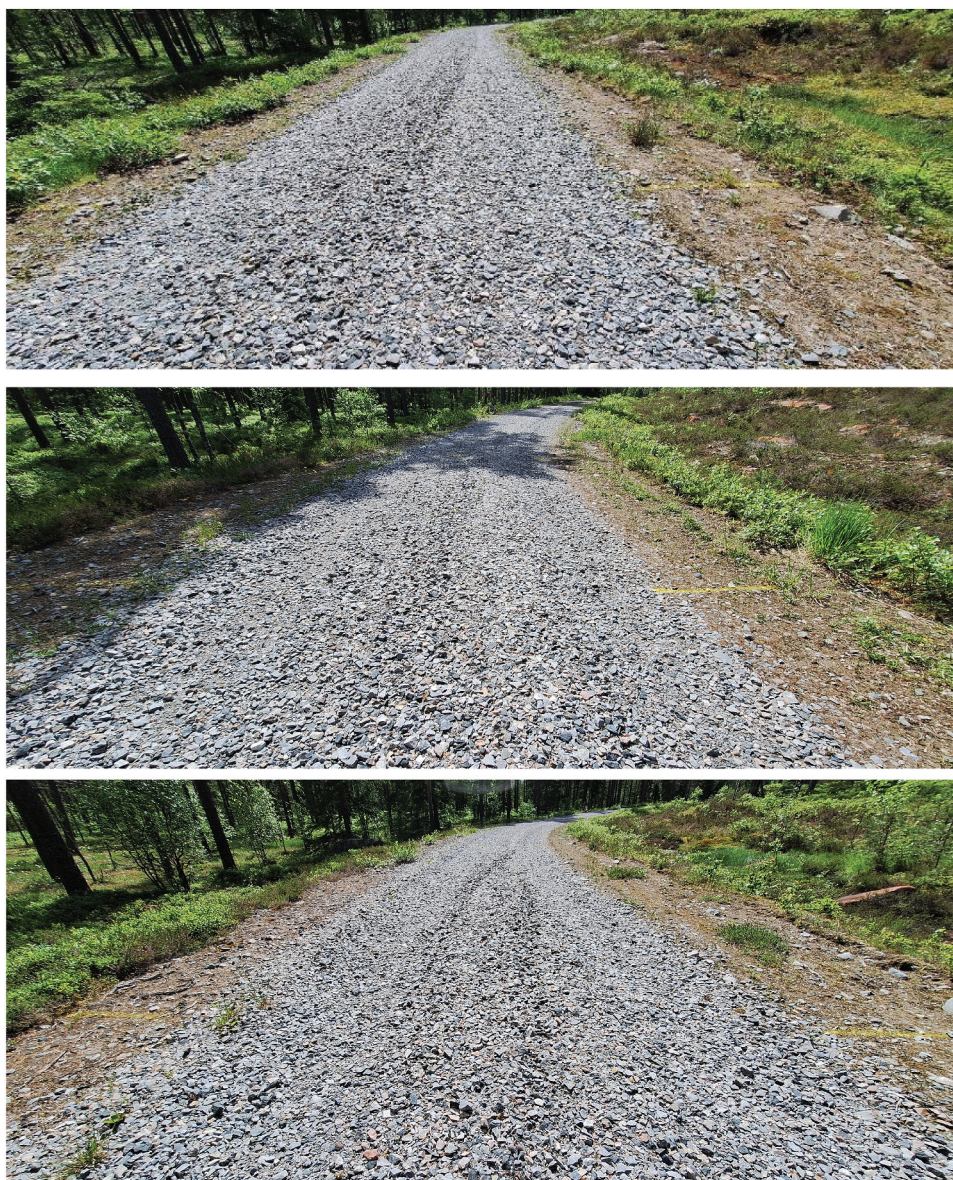
Figure 15. Visual inspection of section 1 (without stone mattresses) in Grängesberg. Photos: Andreas Waldemarson, VTI.
