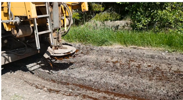
Fig. 4. Stabilization of a selected forest road in Trosa using low environmental impact additives. Photo by Jan Tikkinen, Vumos (Finland).
