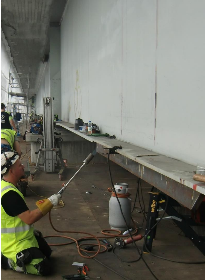
Figure 18. Pre-heating of a longitudinal stiffener before welding. The outer end (near camera) later to be HFMI-treated at the weld toe around the end section (2dm on each side plus at the corner).
