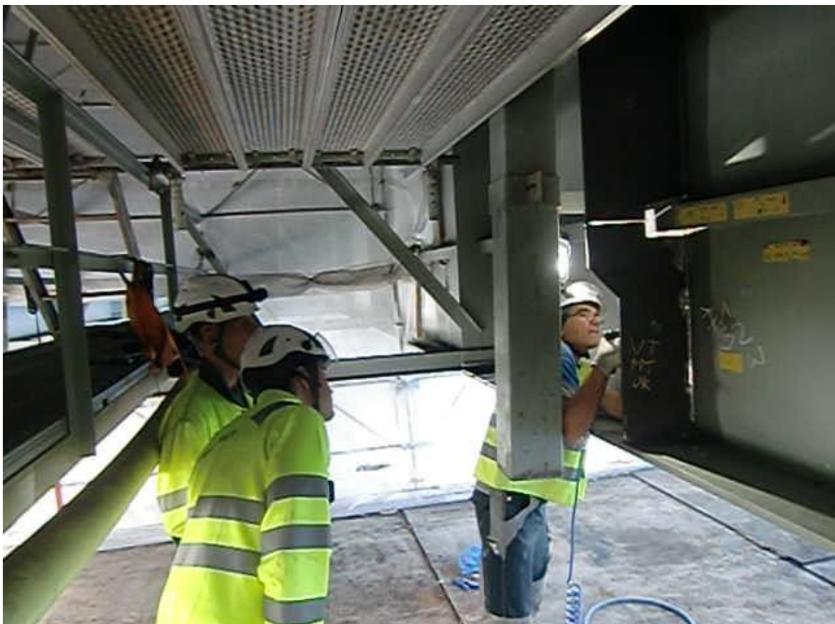
Figure 22. HFMI treatment of a vertical stiffener on the west I-beam of the bridge. The weather protected platform mounted under the bridge gave a good work environment, good access.
