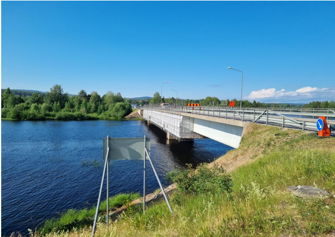
Figure 15. The road bridge in Stöde over the water between Stödesjön and Ede. Note the weather protected platform mounted under the bridge that together with the permanent inspection path between the I-beams gave good work access. Photo taken from north end, I-beams are denominated “west” and “east” beam.
