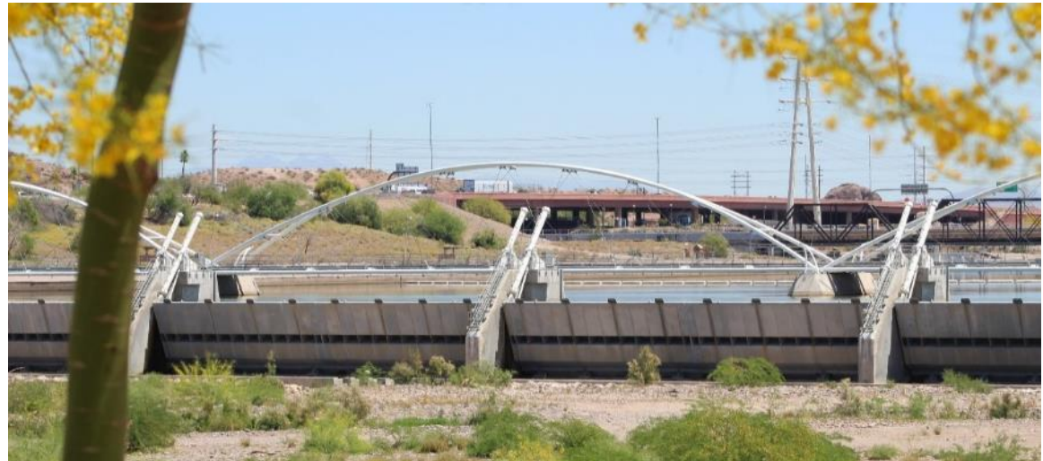
Tempe Lake dam gates
