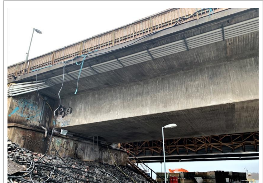
Kalix Bridge: NDT
