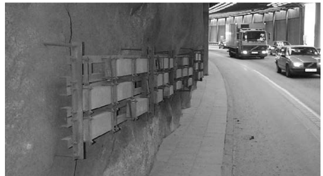
Figure 1 Shotcrete test panels in the Eugenia tunnel, Stockholm. From Nordström (2016).
