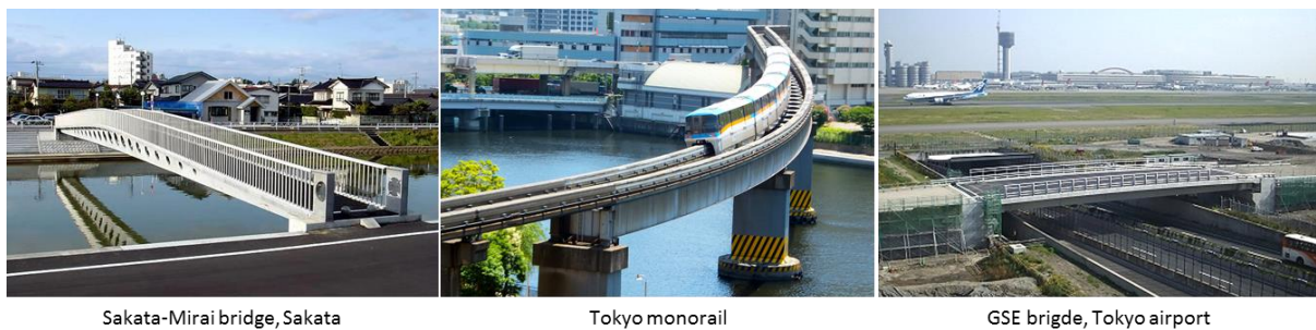
Figure 16 Different types of UHPC bridges produced in UHPC in Japan.
