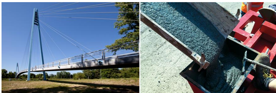
Figure 11 The Elbe pedestrian bridge, Celakovice, Czech Republic ( http://www.heidelbergcement.com )
