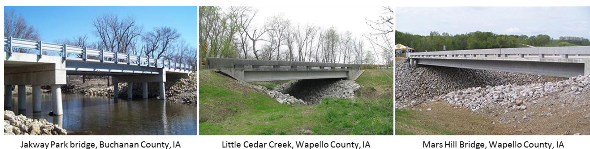
Figure 13 Examples of UHPC application in bridges in USA ( Russel and Graybeal 2013 ).
