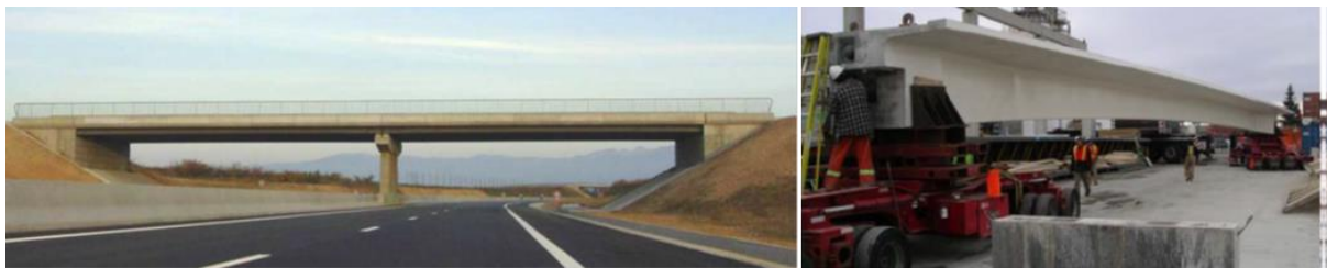
Figure 8 Example of UHPC TT-beam and highway bridge built in France (Lafarge).
