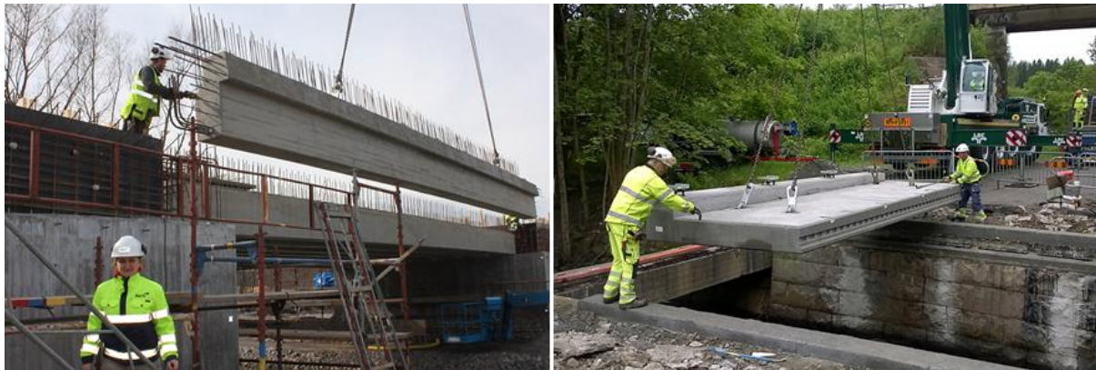
Figure 2 (left) Long span concrete bridge using precast concrete beams and cast in-situ concrete deck bridge developed by A-Betong (right) Short span precast concrete bridge developed by A-Betong. ( http://www.abetong.se ).
