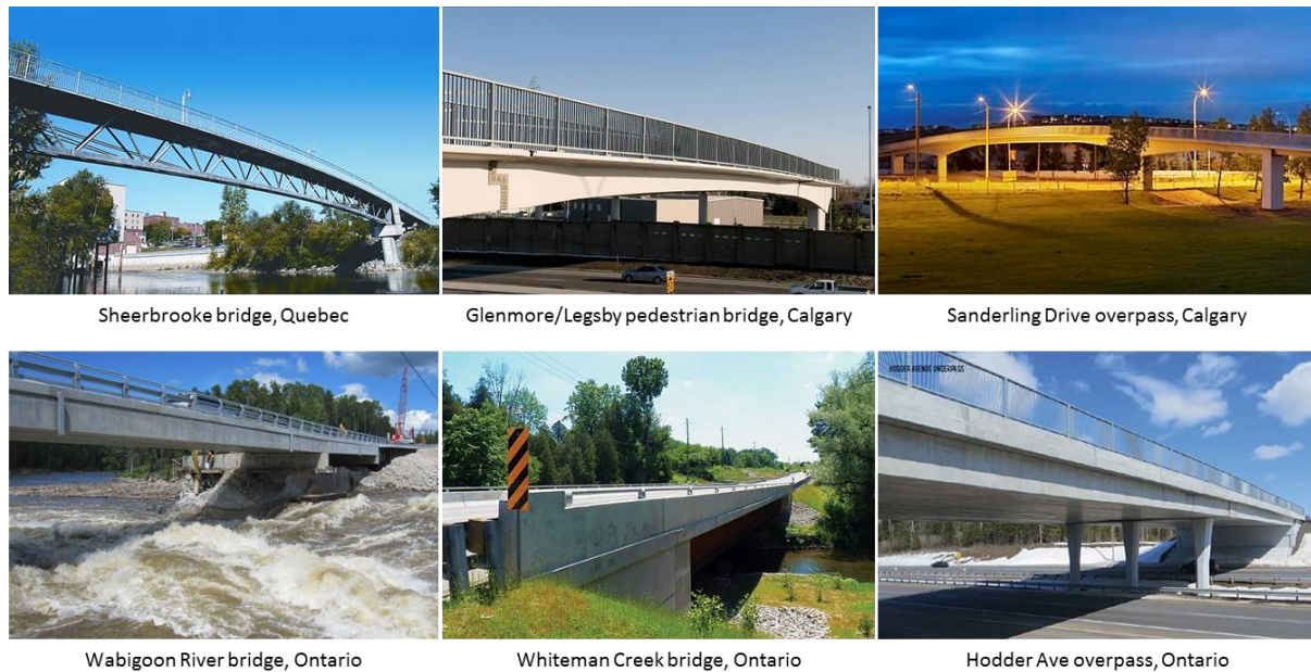
Figure 12 Examples of UHPC application in bridges in Canada ( Russel and Graybeal 2013 ).
