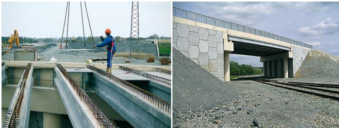
Figure 6 St. Pierre La Cour bridge ( http://www.ductal.com ).
