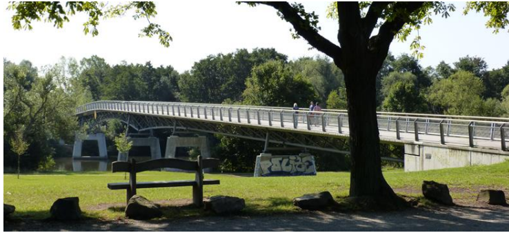
Figure 9 The Gaertnerplatz bridge, Kassel, Germany.
