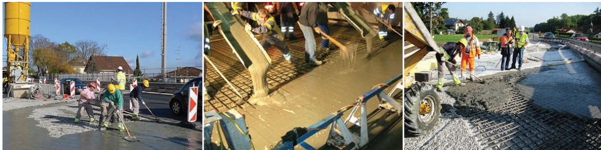
Figure 19 Rehabilitation of bridge decks using UHPC toppings ( Brühwiler and Denarié 2013 ).
