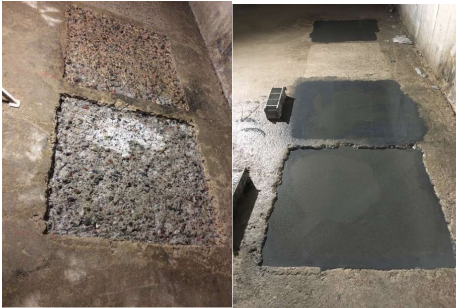
Figure 3-23 Left: two water jetted surfaces, different depth. Right: The three (out of four) surfaces filled with UHPC
