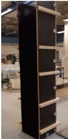
Figure 4-5 Form work, Overlay
