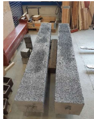
Figure 4-4 Scalled (water jetted) column
