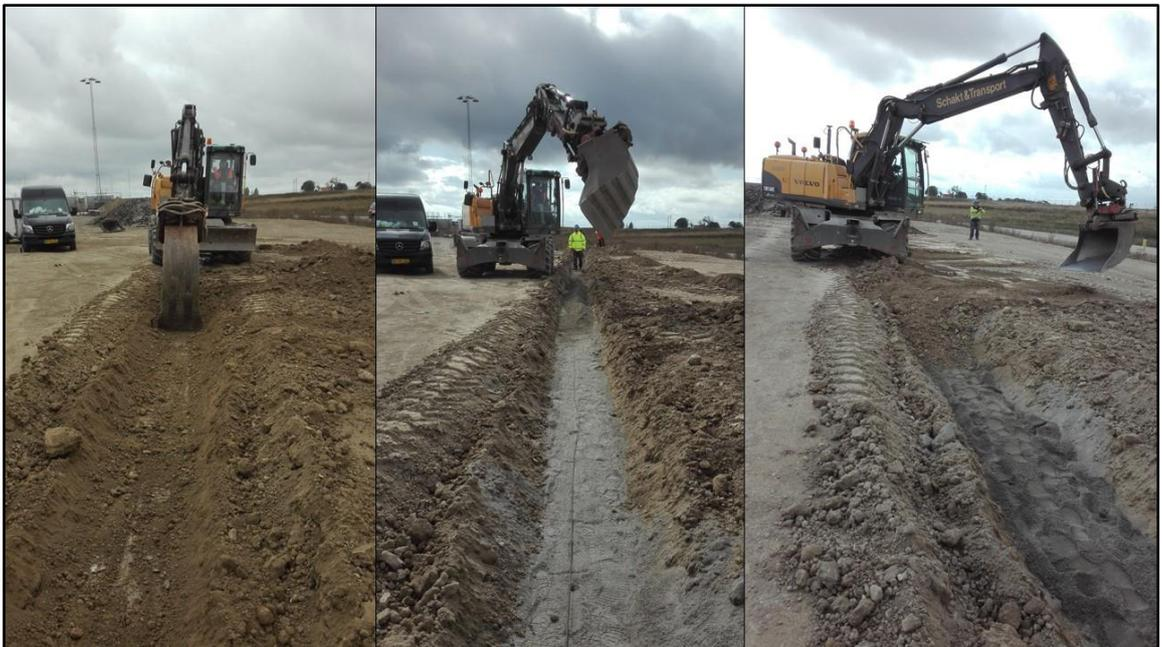
Figure 3.3.2. Pictures of the installation of the fiber optic cable in the ground: left, digging of the trench; middle, cable on top of sand layer; right, backfilling of the ditch with sand and excavated material.
