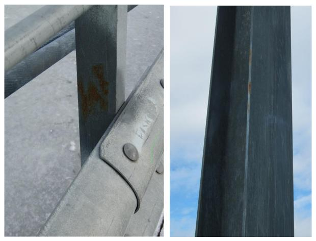
*Figure 58. One or two spots with red rust could be found, these were most probably areas where the coating application for some reason had failed.*
