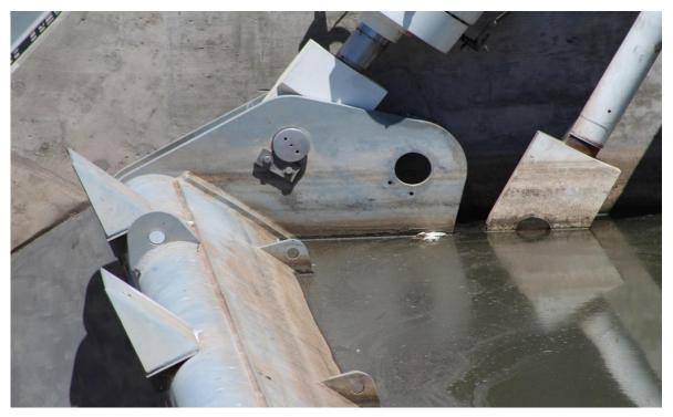
*Figure 28. A picture of the wet side of a dam gate, notice the absence of corrosion around the hydraulic cylinder attachment points.*
