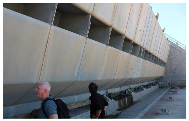
Figure 27. Overview of one out of eight dam gates. The brownish surfaces in the pictures are not rust but have been fouled by running water or dirt from the surroundings.
