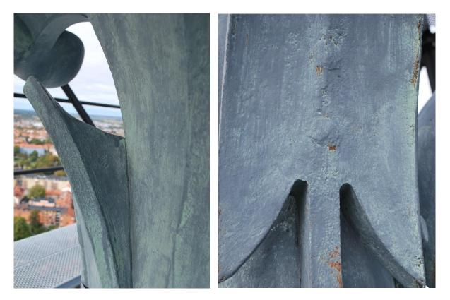
Figure 79. Cast iron ornaments, To the left: a crevice that has been successfully coated without any signs of corrosion. To the right: some under-rusting near edges and rivets/ bolts could be seen.
