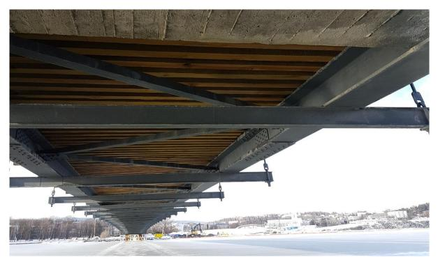
Figure 55. The underside of the bridge. Steel beam girders with support lattice and hanger beams. The distance from the steel structure to the salty water is about 2,5 meters. As there are many crevices and sharp edges on the steel beams, the structure is not optimal for coating
