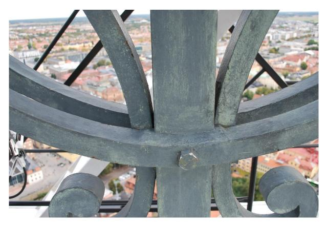
Figure 82. The top of the wrought iron cross, it appears as if the bolt holding the assembly together is made of stainless steel. Probably these parts have been disassembled so that the surfaces in the crevices could be coated, at some point during the early 1970's.
