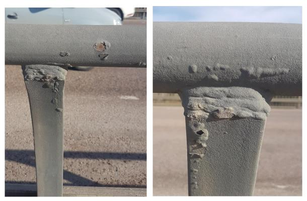
Figure 74. The welds between the fencing poles and the handrail was not optimally prepared. On a few poles some blistering and flaking of the TSZ could be seen.
