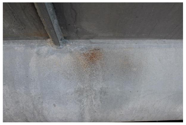
Figure 31. An area with rust spots. This could be a result of poor coverage or dry spray. Or it could be foreign matter from a disc grinder.
