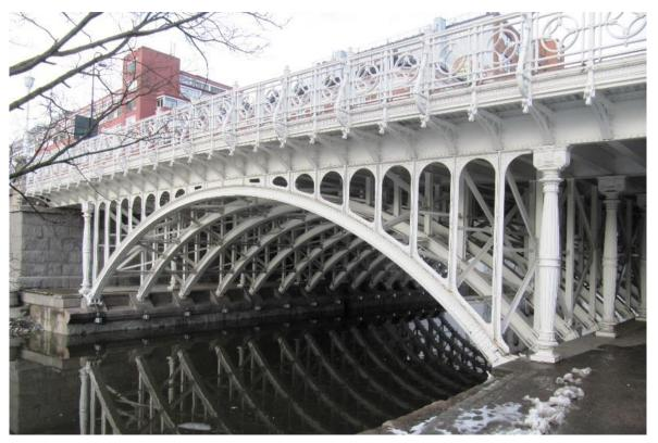
Figure 64. Overview of the Hausmann bridge, the bridge is composed of old cast iron and the center of the bridge is made from modern steel I-beams.
