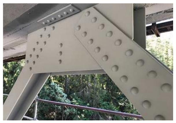
*Figure 45. The coating refurbishments appeared good. All rivet heads had been painted by brush before a final layer of sprayed Zinga was applied. No sags, running or cracking could be found.*
