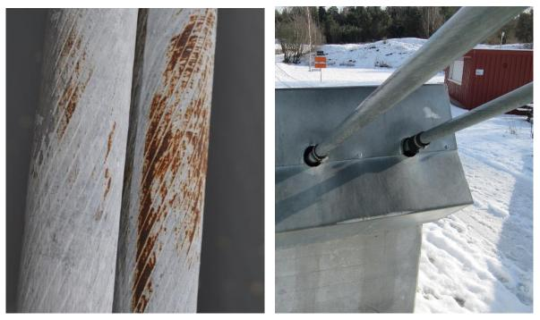
Figure 57. To the left: archive picture of a stay cable after 29 years in service. To the right: Stay cable in 2017, three years after the refurbishment.
