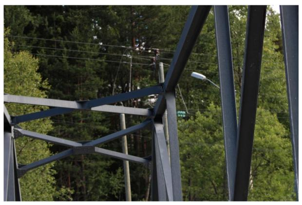
*Figure 47. Granli bru, an overview of the steel structure. The bridge is composed of I-beams connected with riveted steel plates.*
