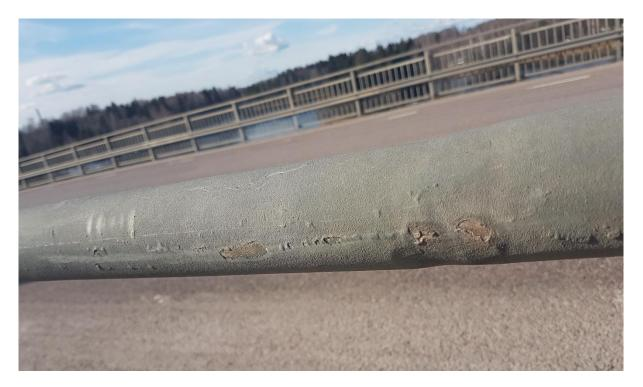
*Figure 75. Mechanical damage on the handrail. Only limited rust creep from the damages was observed.*
