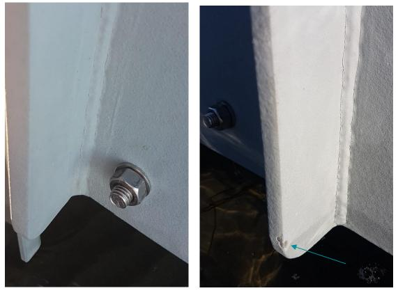
Figure 38. Cracks in the coating along an involute weld seem. It is likely that the cracks penetrate through the first coat but not the coating layer closest to the steel. To the right: A damage in the coating, no corrosion.
