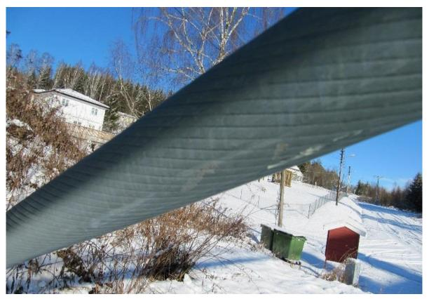
*Figure 63.* A cable near the anchoring fundament. No corrosion was observed on the part of the cables that were accessible during the inspection.
