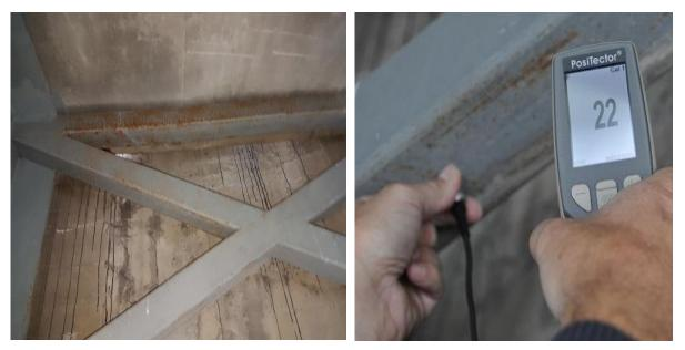
Figure 52. A few surfaces with red rust were found. To the left: the square steel beams were located under a gap in the roadway between the road and the concrete roadway. To the right: The DFT of the square beams was about  $20\mu m$  thick. The breakdown mechanism of the coating appears to be a slow erosion from the outside and in, rather than a through blistering and flaking.
