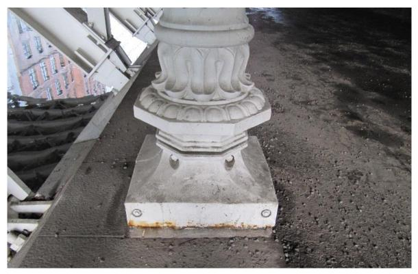
Figure 67. Some rust between the pavement and the cast iron pillars could be seen under the bridge.
