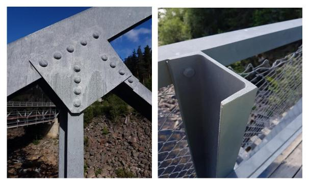
Figure 48. The steel beams of the structure have sharp edges. The design is not optimal for corrosion protection since there are many crevices and surfaces where dirt and debris can collect. No corrosion was observed.
