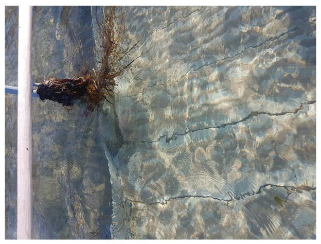
*Figure 35. The ramp can become covered by sand. The lower part of the ramp is subjected to constant abrasion by beach sand moving with the waves.*
