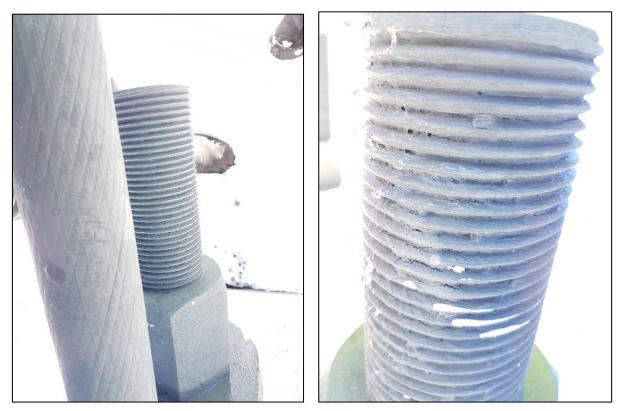
*Figure 62. To the left: cable at the anchoring point. To the right: Coating on a bolt thread at the anchoring point, some pinholes were visible in the thread. There were however no signs of corrosion.*
