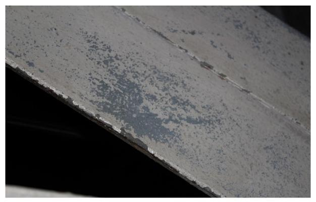
Figure 4. A steel beam in the supporting structure that had been subjected to wear from bypassing visitors. The coating on the edge of the steel beam had been scraped off leaving the underlying steel exposed to the air.
