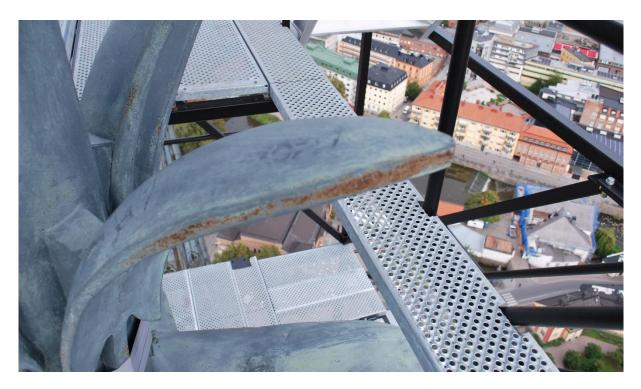
Figure 80. Under-rust on the edge of a cast iron ornament
