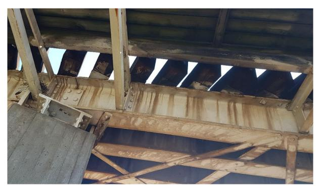
*Figure 86. The brown color is not coming from corrosion but from the wooden sleepers of the train tracks.*
