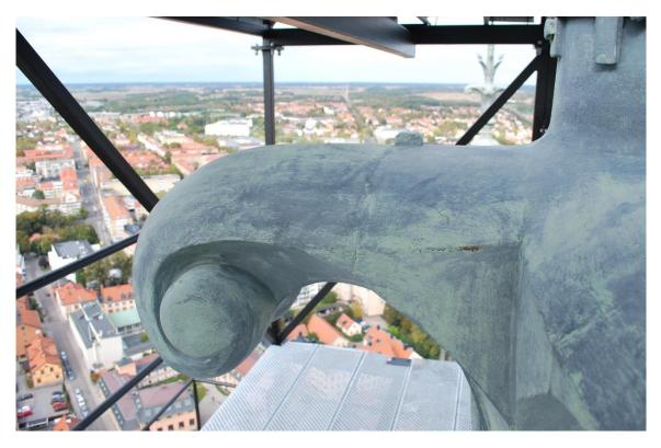
*Figure 78.* An example of an ornament in cast iron, largely an intact zinc coating, a small spot with under rust was visible. The grey chlorinated rubber has deteriorated completely.
