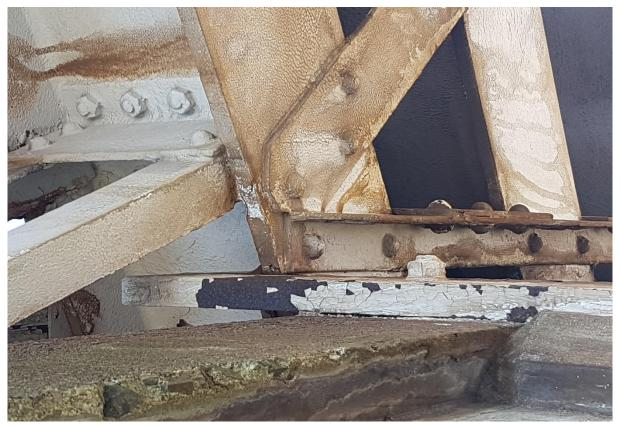
Figure 87. The coating was in some places very thick and had started to flake
