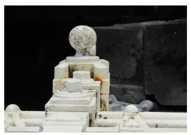
Figure 65. Joint between support arch and fencing post in cast iron. At some joints, discolorations from corroding steel inside crevices could be seen
