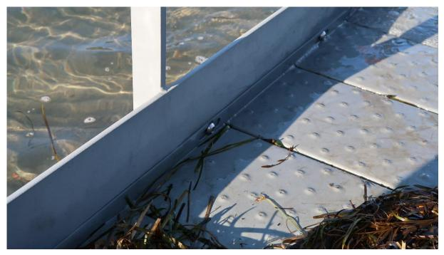
Figure 36. Close up of the ramp floor: there are lots of crevices and the design is not ideal for coating work.
