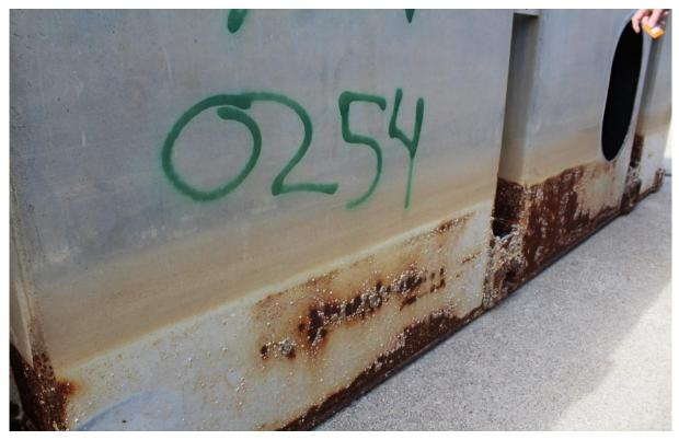
Figure 20. Unit Q0254 Barnacles under the waterline. Intact coating above the waterline
