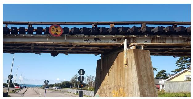
Figure 84. Overview of a railway bridge coated with Eon Coat, the bridge is located near the sea. The coating had started to flake on the main I-beams.
