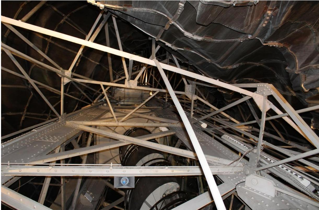
*Figure 2. Overview of the supporting steel structure, light gray in the picture. In the middle of the picture is the spiral staircase leading to the top of the statue. The copper cladding of the statue was black on the inside.*
