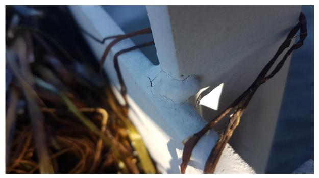
Figure 39. Mudcracking around a weld joining the girder of the ramp with one of the fencing poles.
