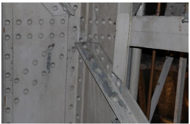
*Figure 3. Supporting steel structure with rivets, the top coat (light gray in the picture) was flaking and peeling off from the underlying silicate (blueish gray in the picture).*
