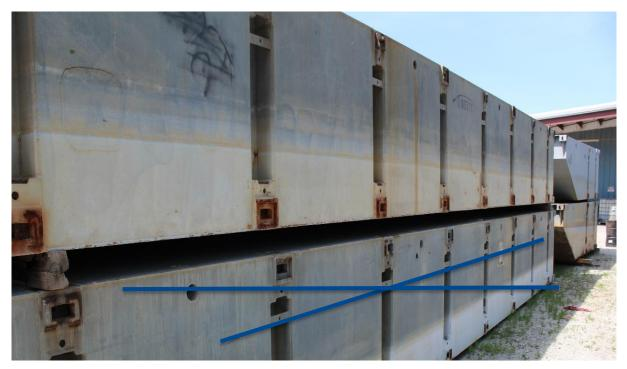
Figure 17. Unit Q155FC, probably manufactured during mid-1990. DFT about 350  $\mu$ m above the waterline and about 260  $\mu$ m below water line, no mudcracking could be found.
