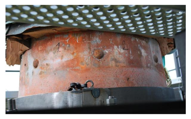
Figure 77. The top of the spire is constructed around a steel cone made from galvanised sheet metal, on the outside it has been painted with red lead linseed oil.
