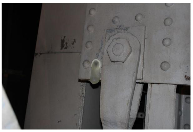
Figure 6. Two Bresle tests were carried out, the amount of soluble salts was equivalent to about 600-800 mg  $Cl/m^2$ . According to the warden of the statue, there had previously been quite a lot of holes in the copper cladding and the high salt content could be a result of rainwater seeping through the cladding. The high salt content on the surfaces could also have been obscured by zinc salts and hydroxides from the silicate coating.
