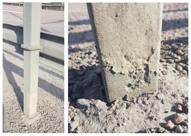
Figure 71. To the left: fencing pole with lower parts coated with epoxy and polyurethane. To the right: Fencing post with completely deteriorated coating, The TSZ under the coating was largely intact, although some spots of red rust had started to emerge.
