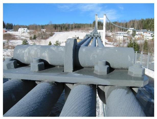
Figure 60. Close up picture of the cable linkages. These parts are not optimal to coat, there are a lot of crevices, sharp edges and areas where it is hard to get good coverage. No corrosion was observed.
