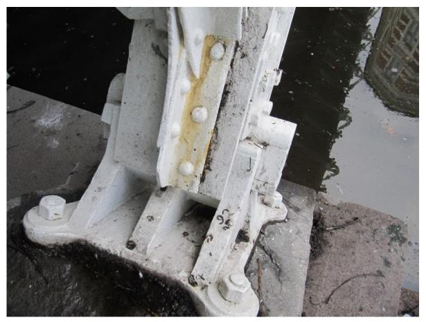
Figure 66. discoloration from crevice corrosion under rivets.
