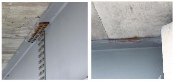
*Figure 53.* A few surfaces with red rust were observed. Unfortunately, these locations were inaccessible for DFT measurements at the time of inspection.
