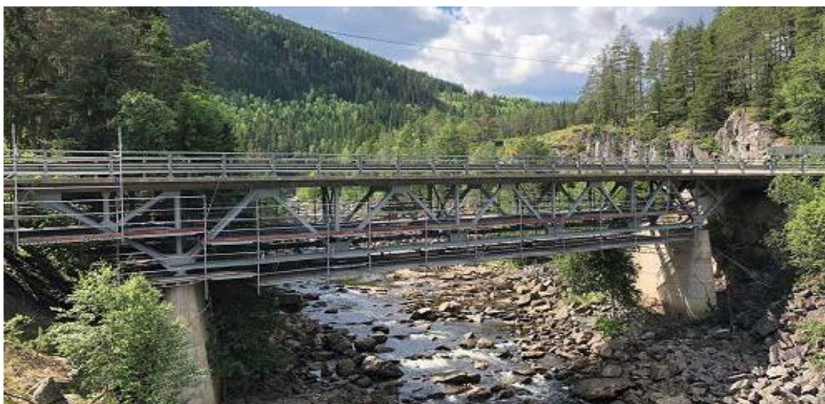
Figure 43. Ro Brua, under the late stages of refurbishment 2018.
