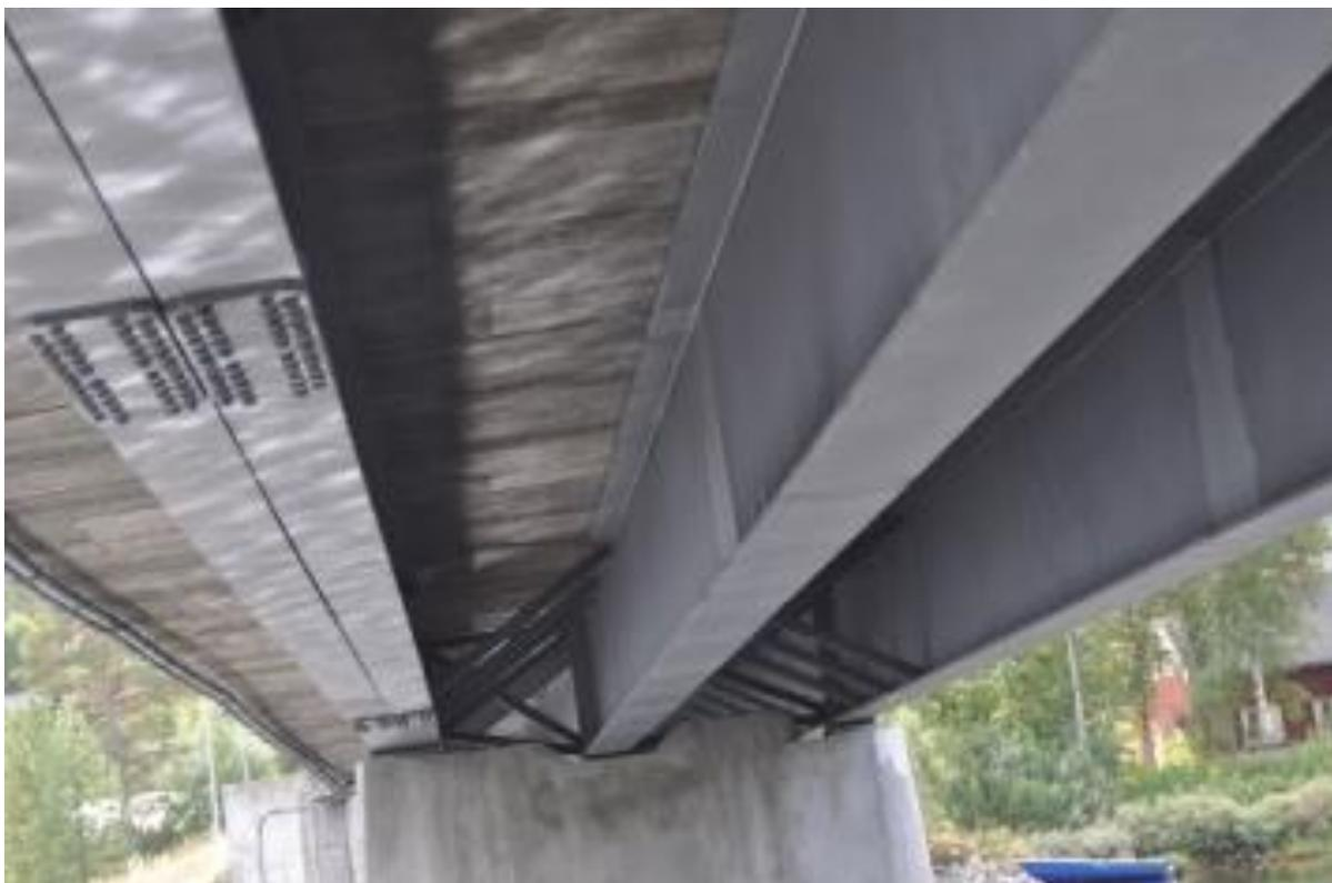
*Figure 51. The bridge is made of three steel beams and a concrete roadway.*
