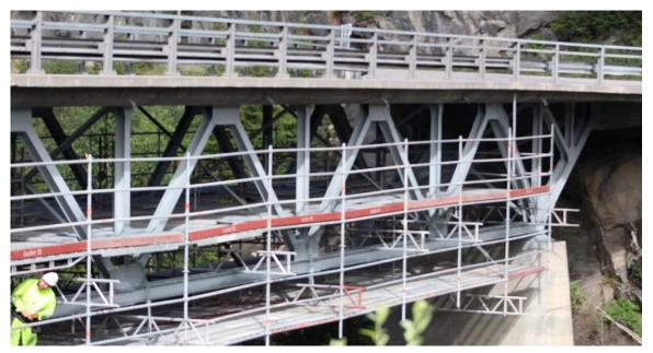
Figure 44. Ro Brua is composed of a riveted steel structure and a roadway of concrete
