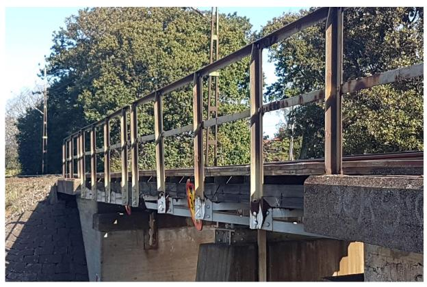
*Figure 85. Corrosion in the joints between the bridge fencing and the support lattice. The picture is from the side facing the sea.*
