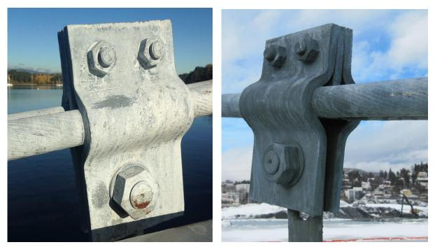
Figure 56. To the left: archive picture from 2014 after 29 years in service. To the right: stay cable attachment in 2017, three years after refurbishment
