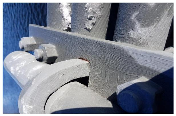
*Figure 61. Clamp joining the cable bundles together. The coating has been applied with a brush, some red-rust had formed inside the crevice between the U-profile and the plate.*
