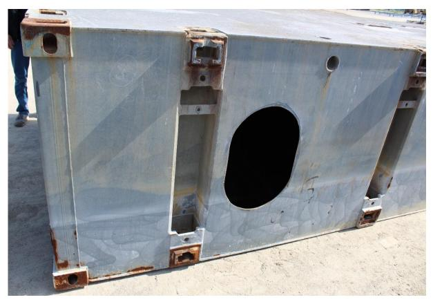
Figure 13. Unit L0 200, manufactured 18 years ago. This unit had been washed with a rotating highpressure equipment, probably to remove barnacles. Most surfaces, edges and welds were essentially free from corrosion. The joints where the units are linked together have started to rust, these areas are however subjected to high mechanical wear.
