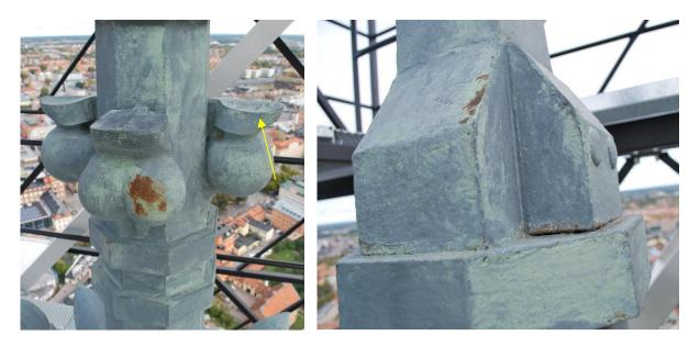
Figure 81. Cast iron ornament, to the left: apparent coating damage on the object before the coating was fully cured. The zinc was about 200  $\mu$ m thick, the coating/ rust layer was about 20  $\mu$ m thick. Notice the year 1974 painted on the right ornament. To the right: the foot of the cross. Some rust on the edges and in the crevice.
