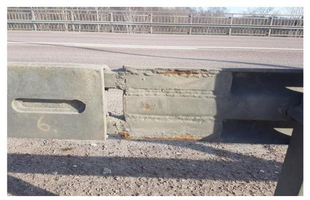
Figure 73. Apparently poorly prepared welds around the expansion joints
