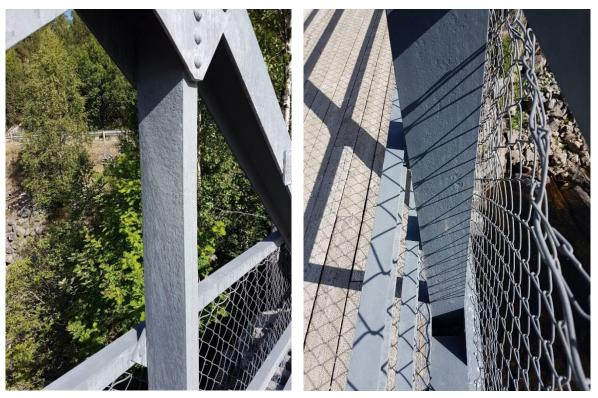
*Figure 49. Surfaces with rough surface profile, probably a result from overcoating steel with rust grade C or D.*
