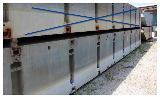
Figure 15. Unit P40 552, manufactured 13 years ago. This module was coated with a mean DFT of more than  $400\mu m$  without any visible mudcracking.
