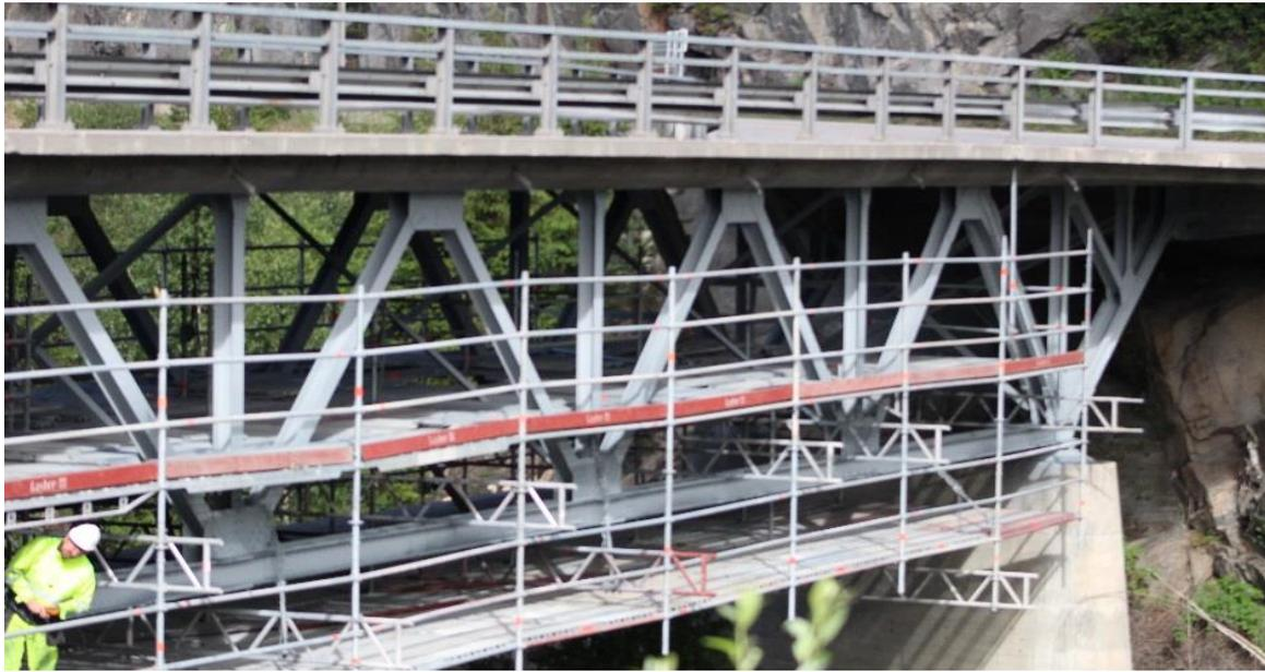
*Figure 44. Ro Brua is composed of a riveted steel structure and a roadway of concrete*
