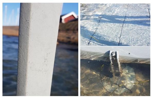
Figure 41. To the left: some craters on a pile for the fencing. To the right: support leg bolted in the girder of the ramp.
