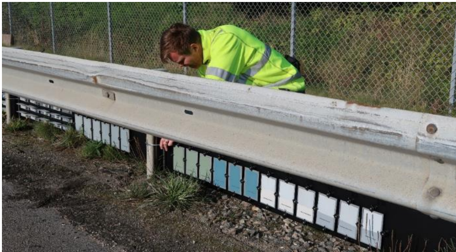
Figure 28. Samples mounted under road fencing at state highway 40,
