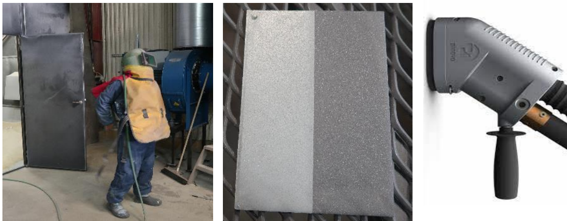
Figure 18. To the left: Blasting in controlled environment is often performed using metallic abrasives. For coating HDG steel it is best to keep as much as possible of the intact zinc and use lower pressures and perform a light blast using inorganic blasting media. In the middle: samples used in this study were blasted to a fine profile with OK grit 55. To the right: vacuum blasting nozzle as depicted at www.pinovo.com . This type of nozzle is suitable for small repairs where dust should be minimized.
