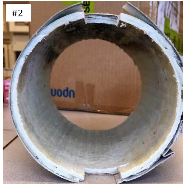
Figure 2. FRP CIPP-liner installed at 2007.
