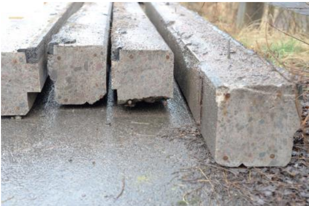
Figure 2. Fragments of the edge beams after cutting
