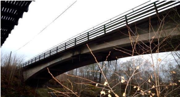
Figure 1. Bridge in Gullspång, Sweden
