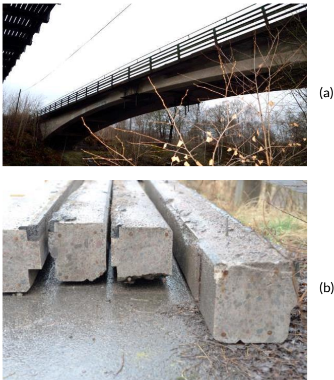
Figure 3 Bridge in Gullspång, Sweden (a) and removed edge beams (b).
