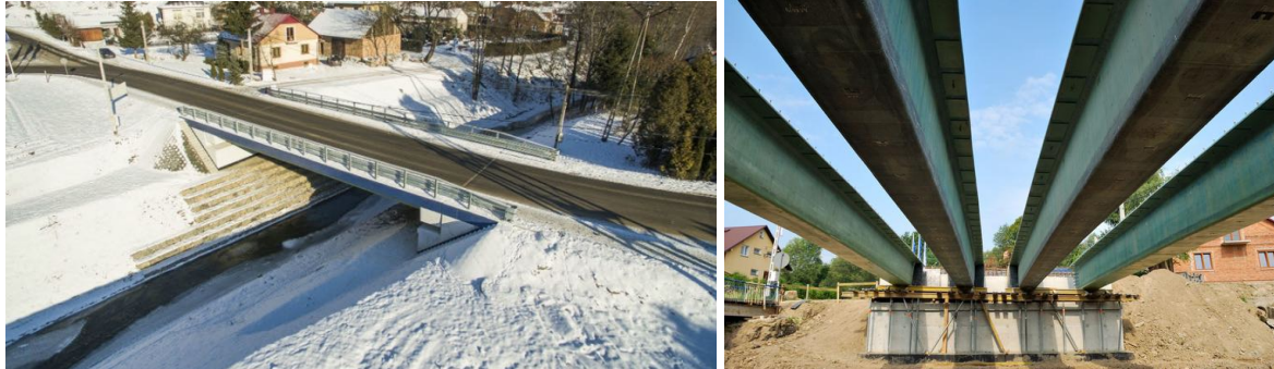
Figure 2 Vehicle bridge with FRP box girders (image source https://polskiprzemysl.com.pl/ , left and https://www.muratorplus.pl/ , right).
