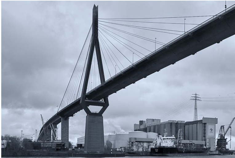
Figure 12 The Köhlbrand bridge in Hamburg, Germany. The main bridge part with the pylons is a cable-stayed bridge, but the access parts are box girder bridges.
