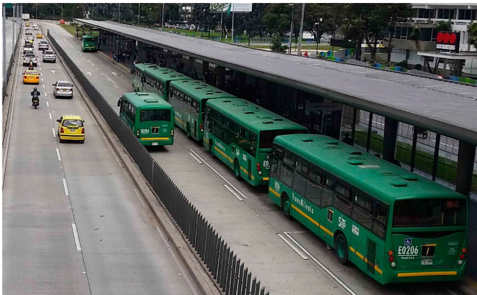
Figure 18 Example of BRT bus station (Colombia)
