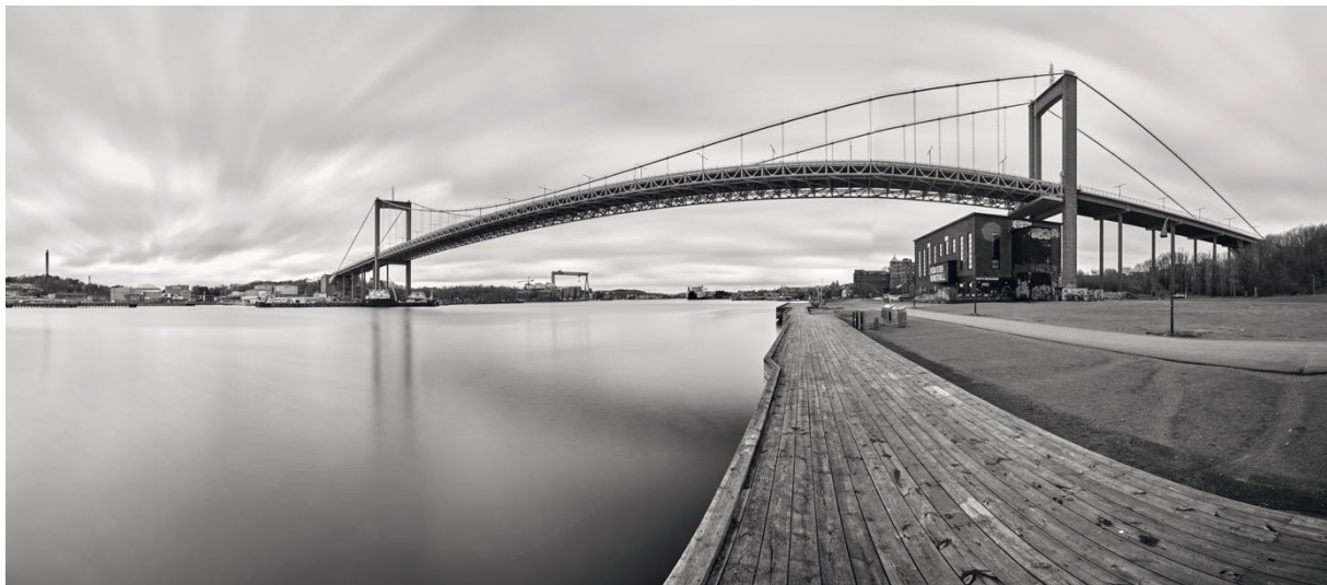
Figure 15 The Älvborgsbron over the mouth of the Göta älv river is a suspension bridge with steel wire cables from the 60s.
