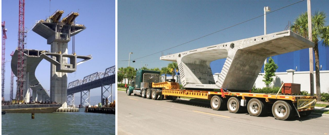
Figure 18 Precast segmental construction in practice. Images from www.asbi-assoc.org .
