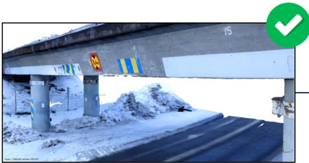
Photogrammetry scanning: Point cloud 3D model of exterior
