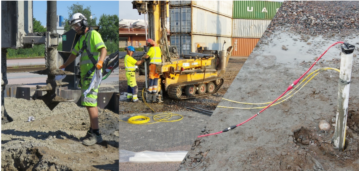
Figure 1 Documentation of the field installations and measurements: mixing tool with 80 cm diameter (left), installation of slotted PVC-pipe (middle) and installed ERT-cable (right).
