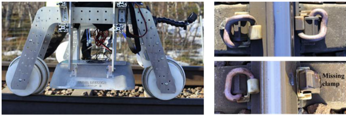
Figure 8. (a) Lindometer measurement system setup, (b) e-clip fastening system, intact and with a missing clamp.
