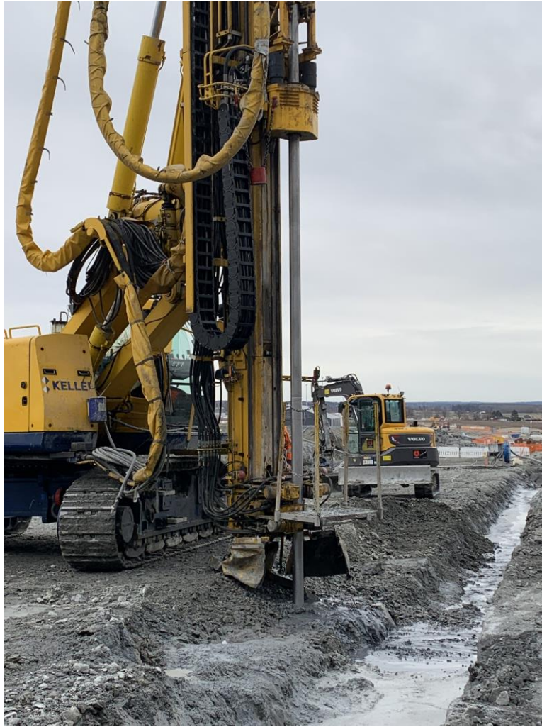
Figure 35 Jet grouting machine inserting steel casing
