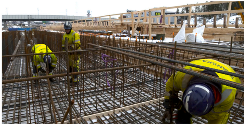
Fig. 1. Manual reinforcement installation in progress.
